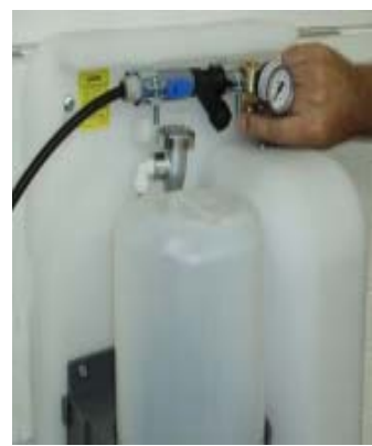
9. Turn on water supply valve. Adjust pressure regulator.
