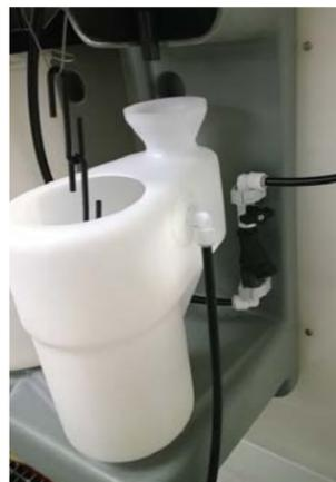
6. Remove plug from overflow port and install other fitting into threads and run tube to your floor drain in the case of an overflow situation.
